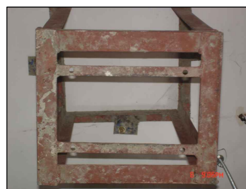
CABLE SUPPORT STRUCTURE
