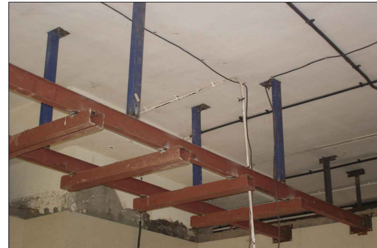
REFERENCE IMAGE - CEILING GRID STRUCTURE
